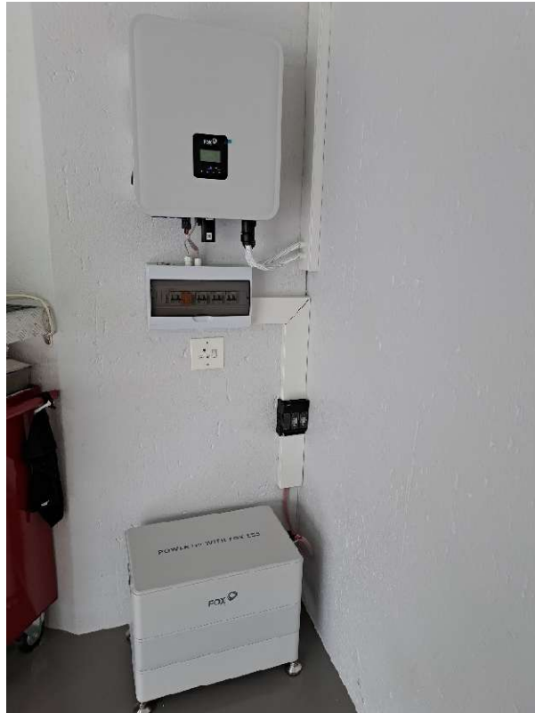
Fox 10.5kW inverter & 12.3kWh battery
